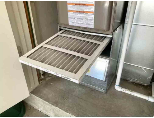
HVAC Filter Placement
