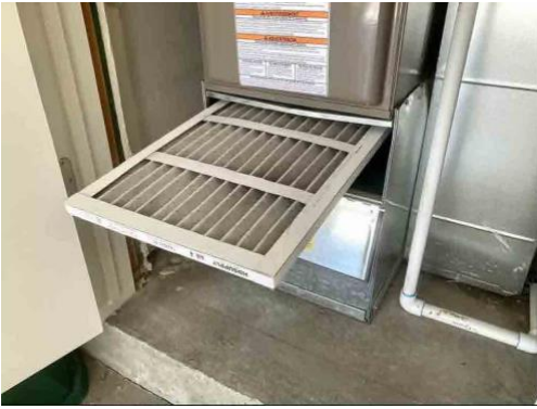
HVAC Filter Placement
